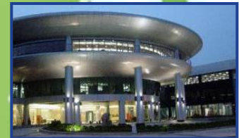
China Technology Center Shanghai, China
